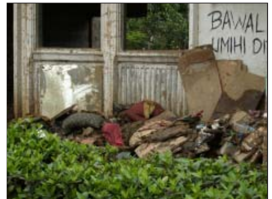
Debris rests alongside a home.
